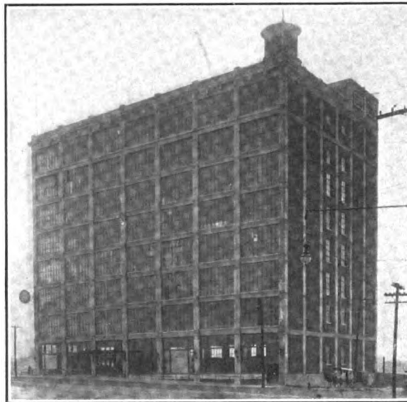
Fig. 2—Exterior view of the building, showing the modern tile and glass construction
